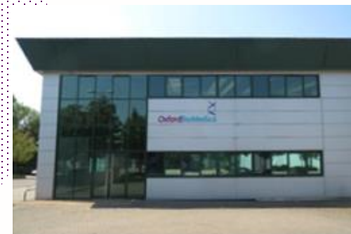
Yarnton (GMP4) API manufacturing facility
