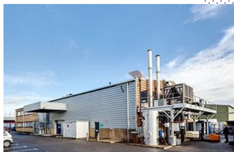
Harrow House (GMP1/GMP2/GMP3) Fill & Finish API manufacturing facility
